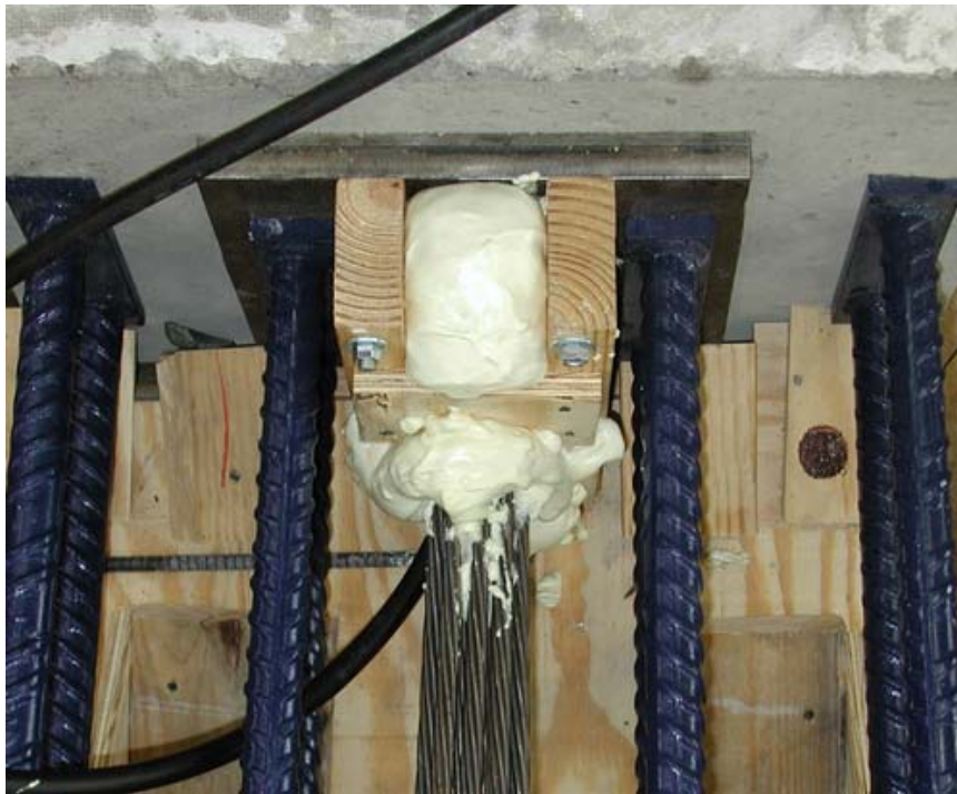
Figure 3-16 Completed Final Foaming
