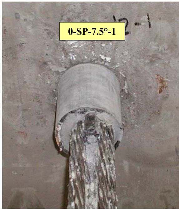
Figure 4-19 Live End of Specimen 0-SP-7.5°-1 after Testing
