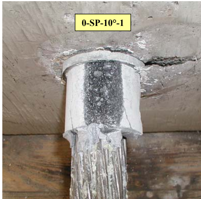
Figure 4-14 Live End of Specimen 0-SP-10°-1 after Testing
