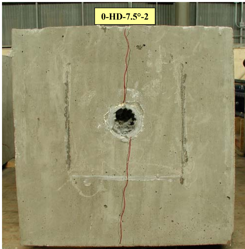
Figure 4-72 Photo of Specimen 0-HD-7.5°-2 after Testing
