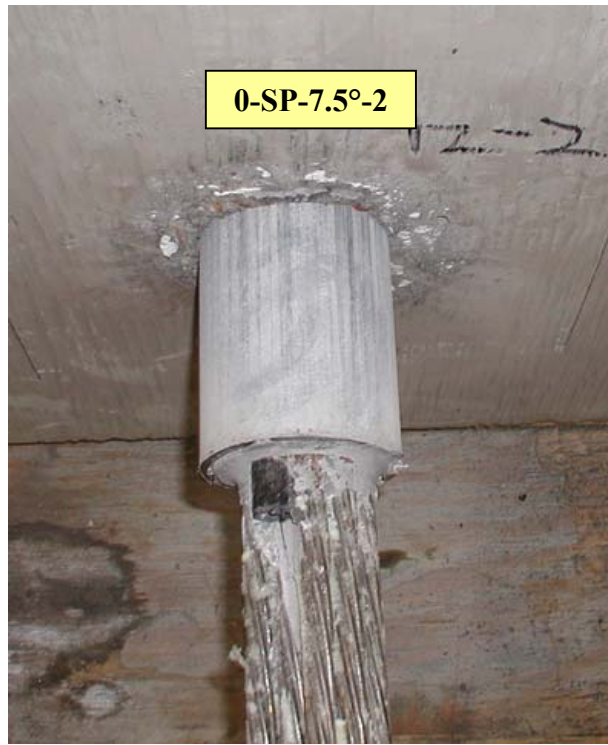
Figure 4-22 Live End of Specimen 0-SP-7.5°-2 after Testing
