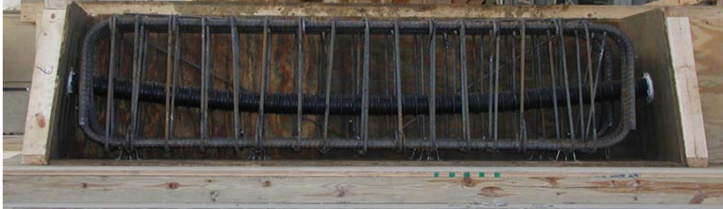
Figure 3-8 Assembled Specimen Cage, Duct, and Formwork
